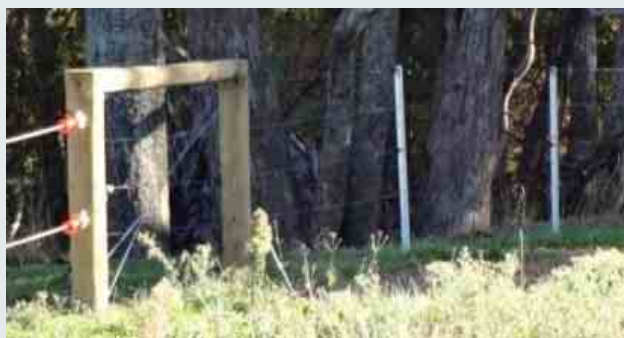
Figure 7.12 – Pine posts at 50 m spacings with steel pickets every 3 m, four plain wires including two electric
