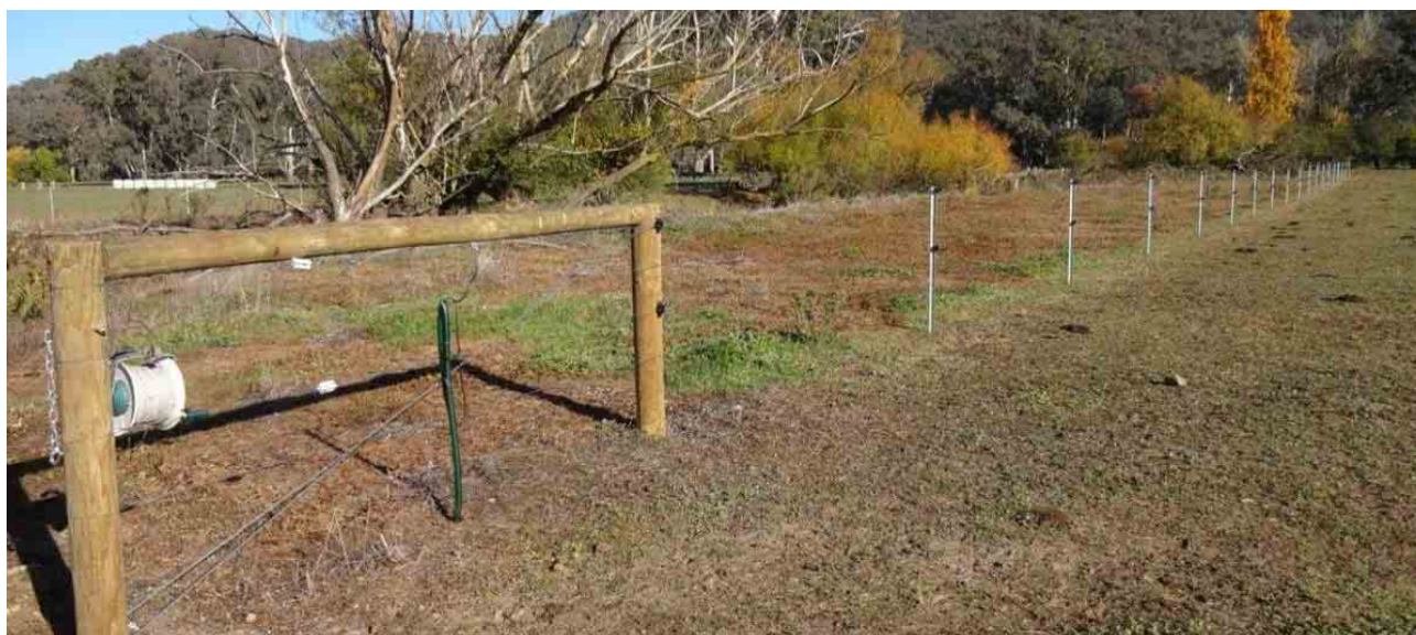
Figure 7.11 – Full-length sacrificial fence
