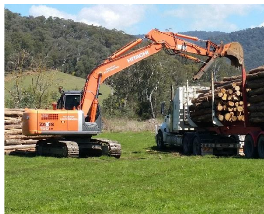
Figure 2: Timber piles destined for the Little Snowy Creek being unloaded onsite
