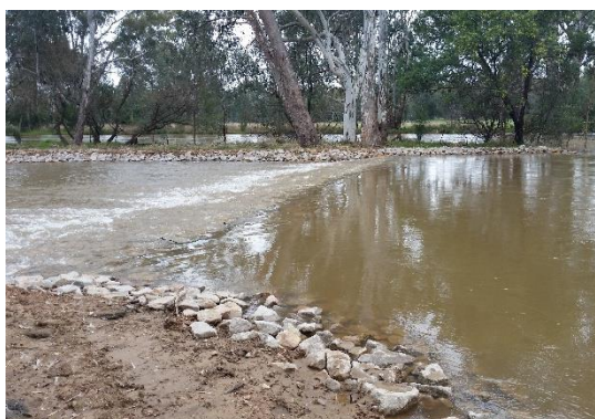
Figure 1: Markwood Breakaway rock chute overtopped with water late Winter 2017
